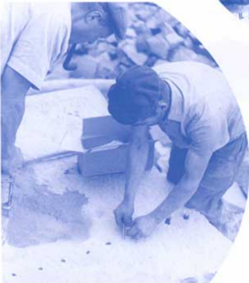
Cutting of granite head with 22 x 115 wedges
